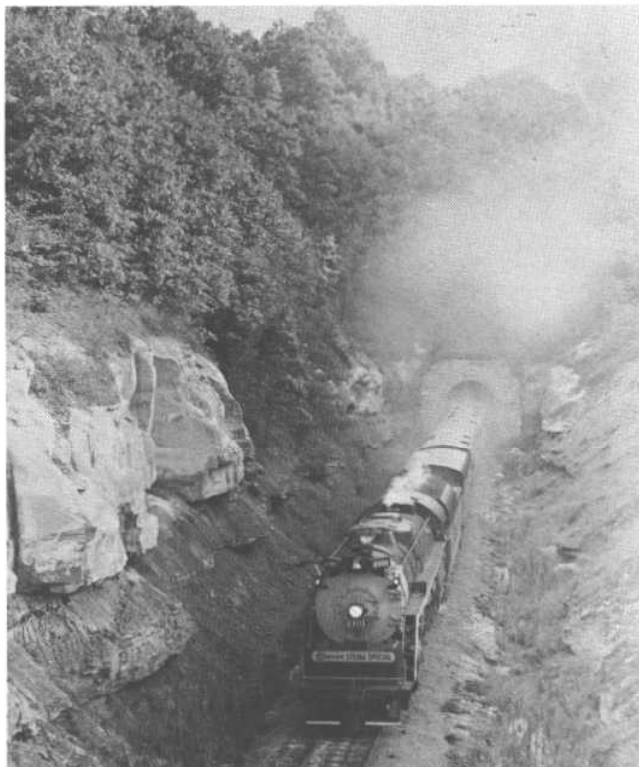
Out of Princess Tunnel on the Lexington Subdivision, August 27, 1977. Photo by Susan Young.
