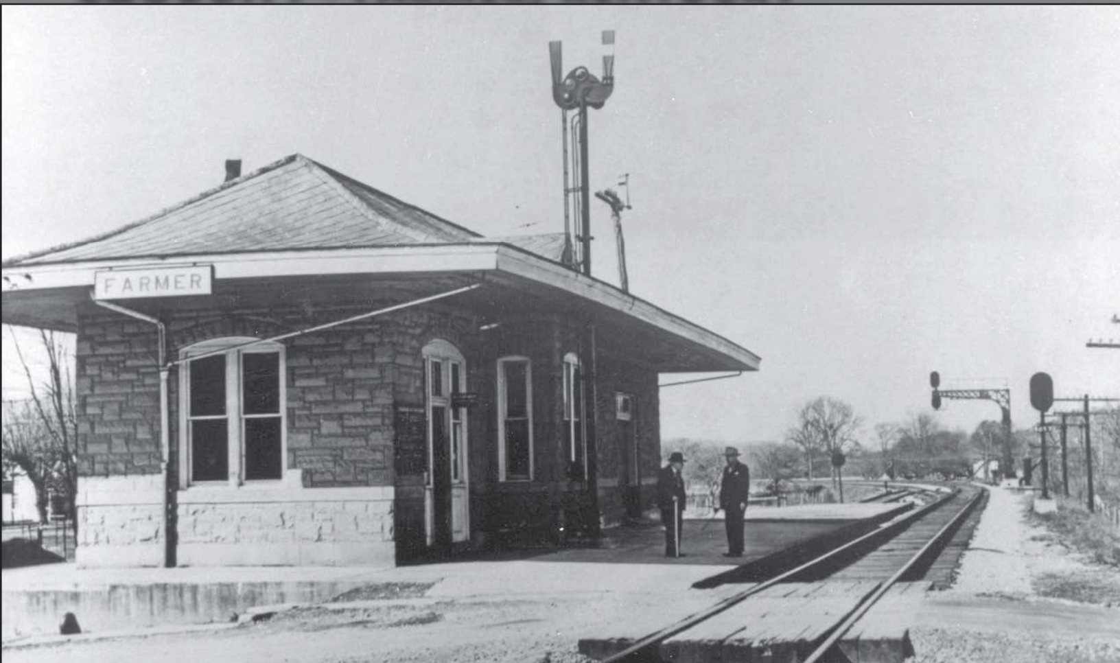
C&O depot building at Farmer, Ky. was built of locally quarried Kentucky Blue Stone in 1911. Here it is about 1950. (C&OHS Collection, COHS 475)
