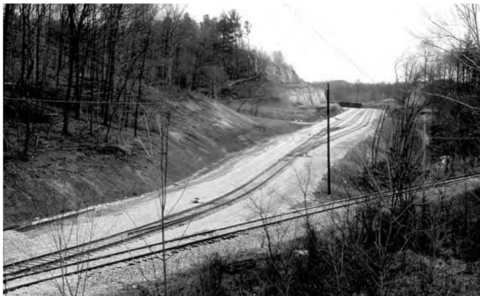
New CSX spur to Enviro Solutions garbage facility at Princess, Ky., on March 19, 2007. This view is from the US 60 bridge.
